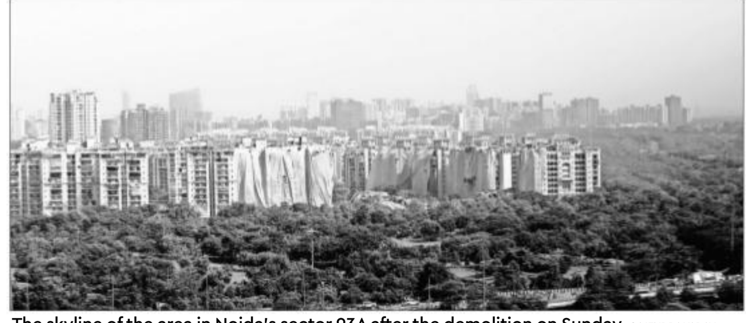
The skyline of the area in Noida's sector 93A after the demolition on Sunday. GAIJENDRA YADAV
